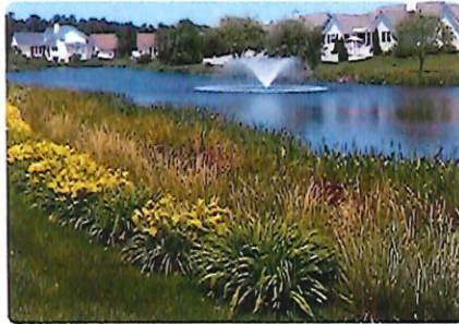
SWM POND WITH AERATION FOUNTAIN
